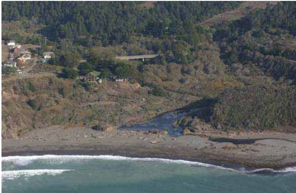
Figure 1. Greenwood Creek Bridge, State Highway Route 1, at Elk, California.
