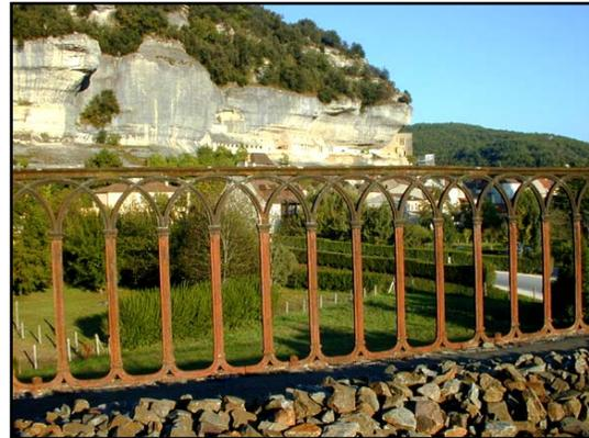
These railing are on bridges in France and are of cast iron. Alternative materials could be used, although cast iron would be structurally adequate for pedestrian railings.
